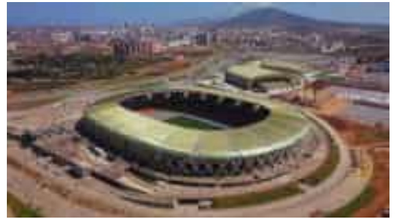
Figure 92 : complexe Mouloud Hadfi
