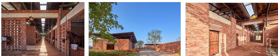
Figure 59 écurie (source : https://www.archdaily.com/870751/equestrian-center-in-luxelakes-eco-city-chengdu-wide-horizon-investment-group )
