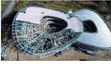
Figure 99 :Charpente en acier Source : www.guardianglass.com
