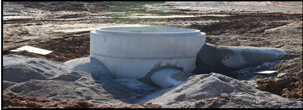
Figure I. 11 Regard de jonction [22]
