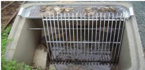
Figure I.6 : Grille manuelle [26]
