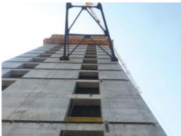
FIGURE 1.3: THE COUPLED SHEAR WALL CORE OF A MULTI-STOREY BUILDING (CARY KOPCZYNSKI&CO.BELLEVUE, WA).
