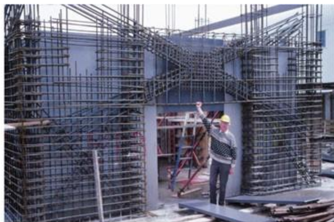
FIGURE 2.6: PROFESSOR TOM PAULAY WORKING ON THE DIAGONALLY REINFORCED COUPLING BEAM IN THE CORE WALL OF CHRIST CHURCH GENERAL HOSPITAL (COURTESY OF J.I.RESTREPO).
