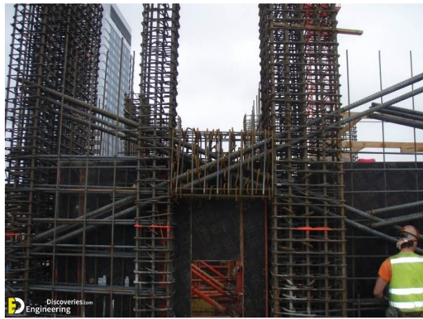
FIGURE 1.1.12: RCC COUPLING BEAM DESIGN AS PER ACI
