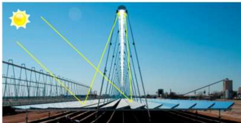
Figure I-9 : Centrale miroir Fresnel [18]
