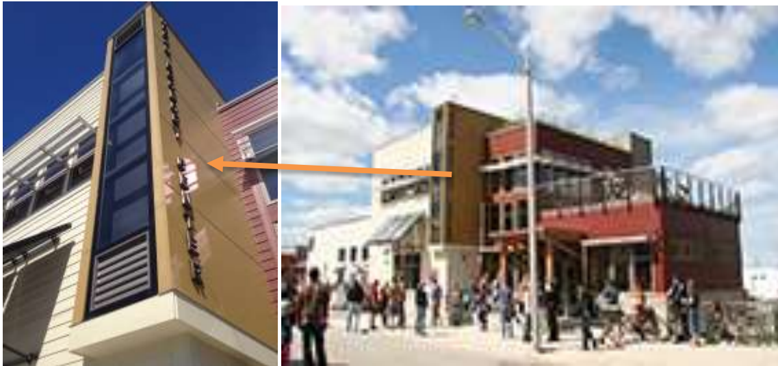
Figure I.7: Solar chimney MENOMONEE VALLEY 3700 W Pierce St Milwaukee, WI 53215, united states [10]
