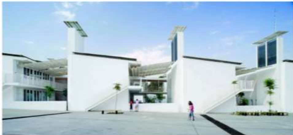
Figure I.23: The coupling of passive systems and a solar chimney [50]
