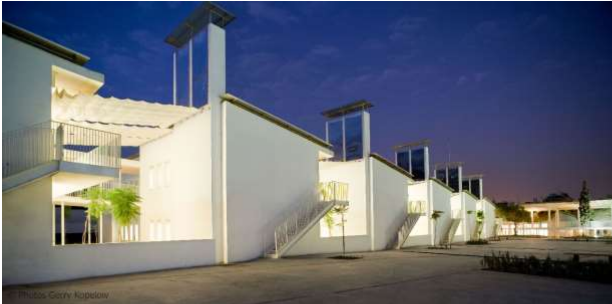
Figure I.19: Traditional ventilation and cooling techniques with solar chimneys and wind catchers in a Damascus School [45]
