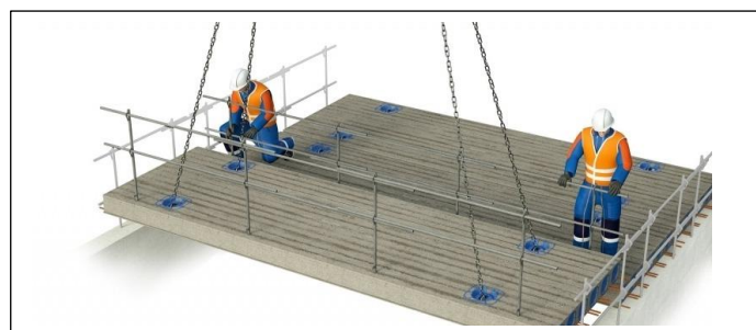
Figure 73: dalle alvéolée: Source: google image
