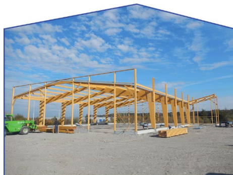
Figure 63: charpente lamellée-collée 87
