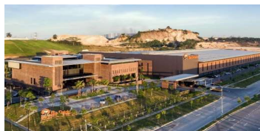
Figure 47:Siège social Big Dutchman Agriculture Source : https://www.archdaily.com/905047/big-dutchman-agriculture-headquarters-and-warehouse-nwka-architects-sdn-bhd
