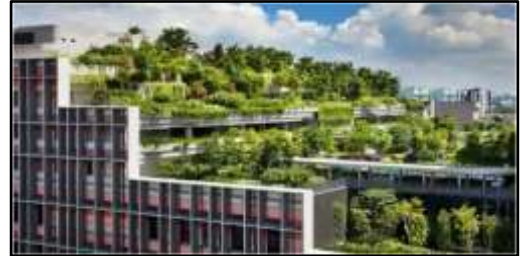
Photo 12 : Architecture écologique (source : https://architecture-ecologique-cest-quoi/ )
