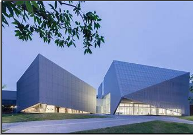
Figure 46 : Miura Showroom Source 8 : www.archdaily.com
