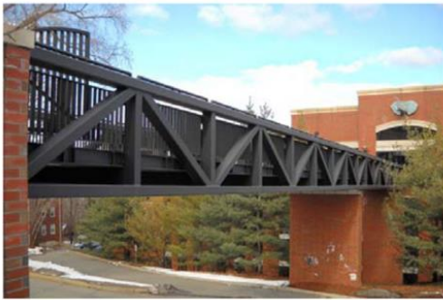
Figure II-8– Passerelle de Dowling Hall [86]
