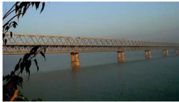
Figure II-9 – Pont de Saraighat [87]
