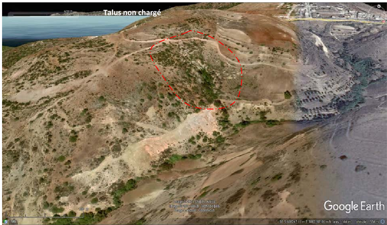
Figure 4.12 : Talus non chargé (Google Earth) [20]
