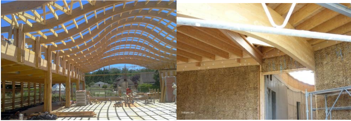
Figure 70 : ossature lamellé collé
