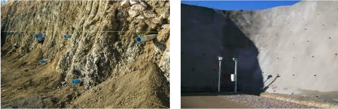
Figure 1.2 System de drainage
