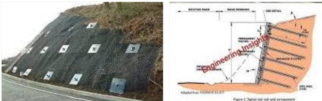
Figure 1.3 Technique de boulonnage
