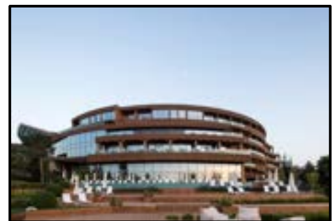
Figure 66: Eskişehir hotel and Spa
