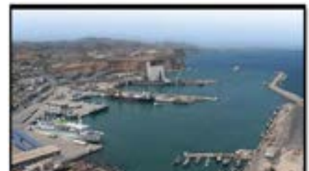
Figure 11: le port de ghazaouet Source : Google image
