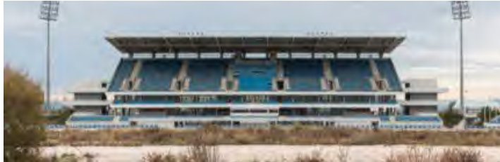
Figure 7. Abandoned Athens Olympic 2004
