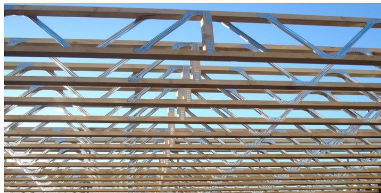
Figure 9: Poutres hybrides acier-bois [65].
