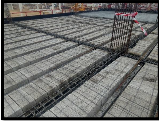
Figure 96 dalle en corps creux
