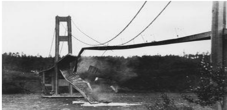
Figure I-8 : Tacoma Narrows Bridge [8]
