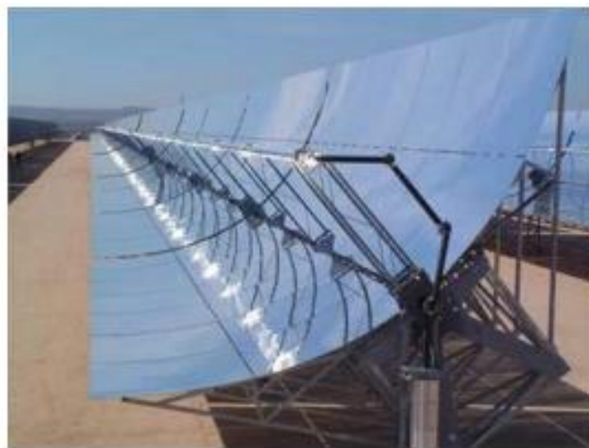
Figure I.11:Cylindrical-Parabolic Collector
