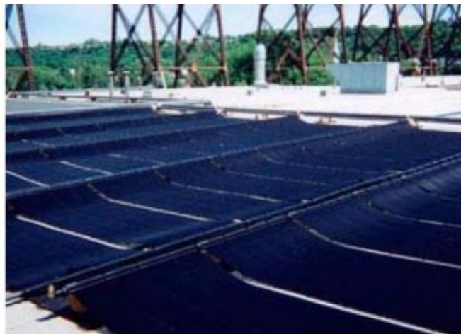
Figure I.8: Unglazed Flat-Plate Collectors
