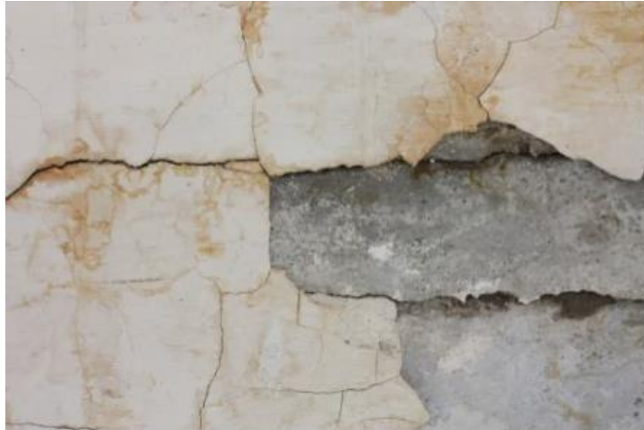
Figure 1. 23: alcali-réaction [33]
