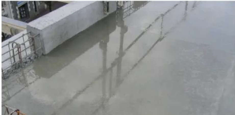
Figure 1. 11: ressuage de Béton [3]
