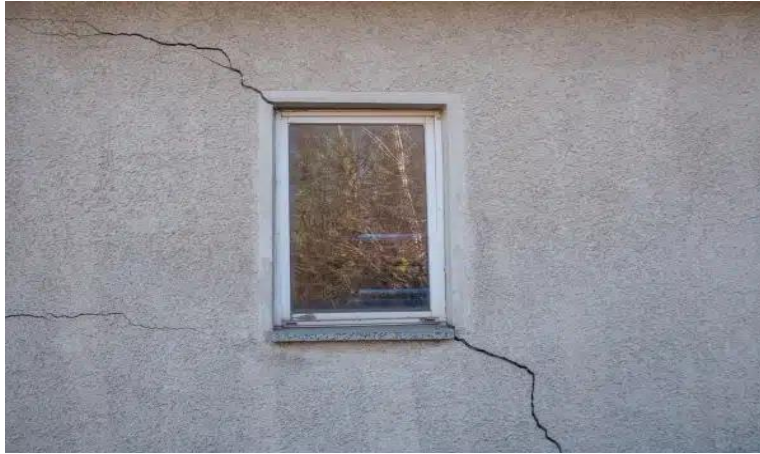
Figure 1. 6: fissure en moustache [5]
