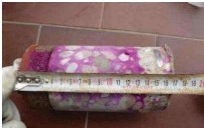
Figure 3. 8: carbonatation sur carotte [12]
