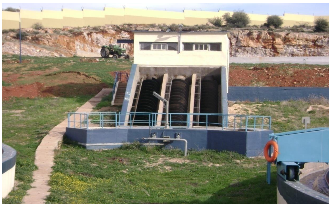
Figure 31: Vis de recirculation
