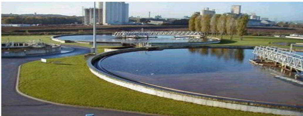
Figure II. 10: Décantation secondaire [17].
