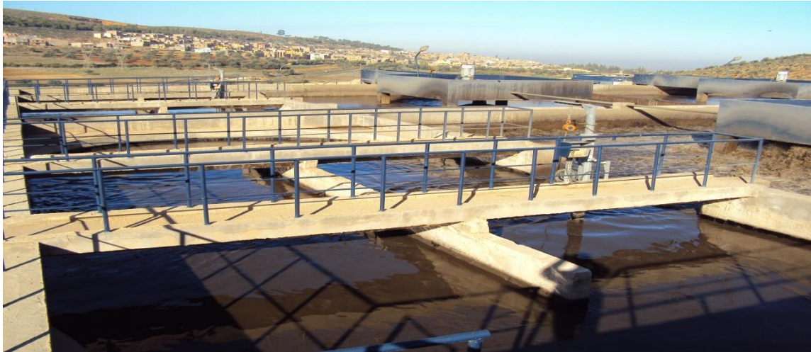
Figure IV. 9: Bassin de nitrification dénitrification [53].
