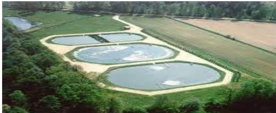
Figure II. 4: Lagunage aéré [17].
