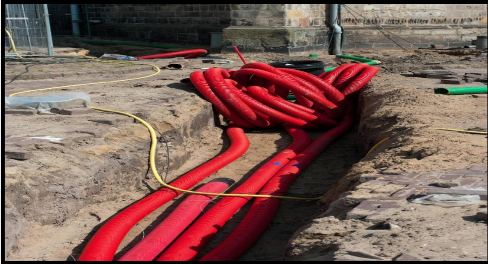
Figure II .2 : Les Câbles souterrains. [II.8]
