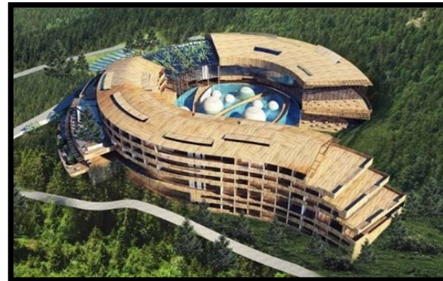
Figure73: Eskisehir spa & thermal hôtel Source: https://i.pinimg.com/564x/9c/3e/5c/9c3e5c407af3ce93c84c2ae2c2f678bd.jpg
