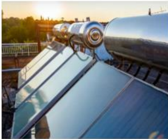
Figure I.1: Chauffe-eau thermosiphon monobloc
