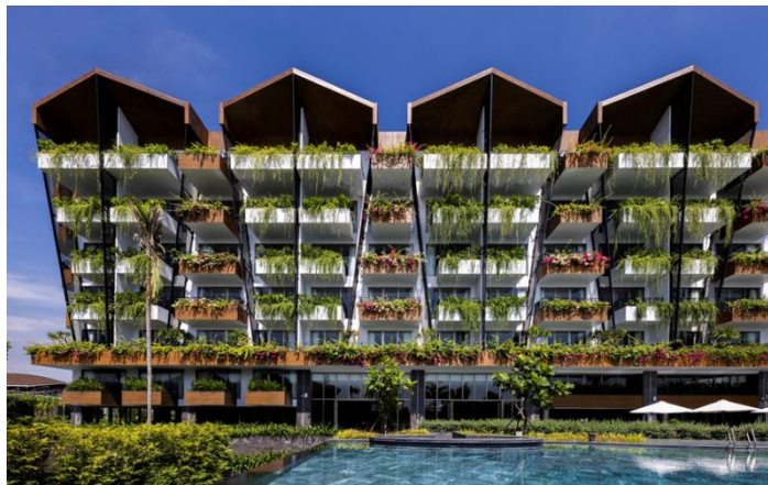
Figure 85. Facade bellerive resort
