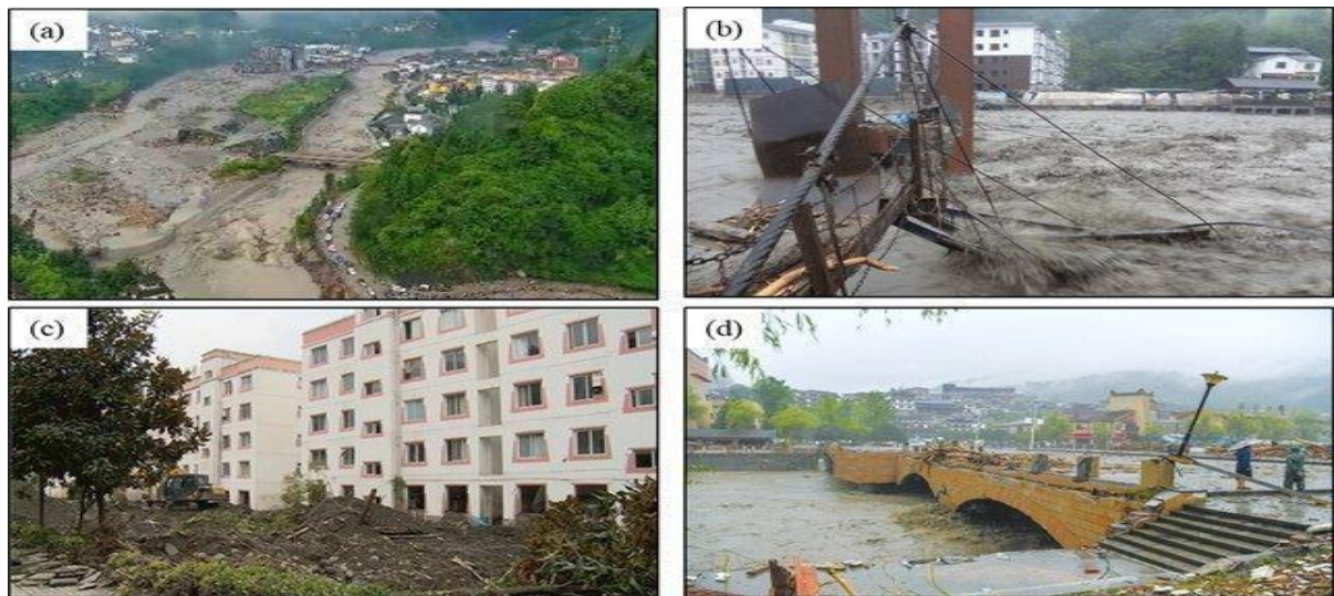
Fig 2.4 Damage caused by flash floods in Wenchuan, china (Jin et al., 2023)
