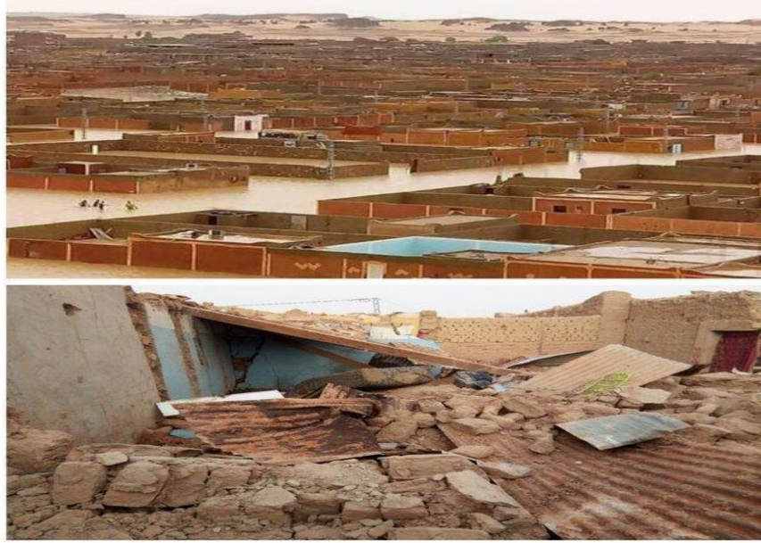
Fig 2.7 flood damage in In Guezzam city in August 2018(Madi & Bidjaoui, 2024)
