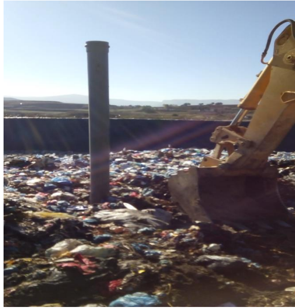
Figure 17 Tube de biogaz
