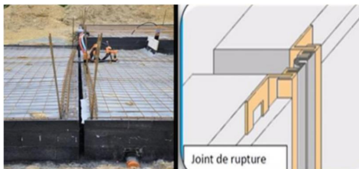
Figure 66: joint de rupture
