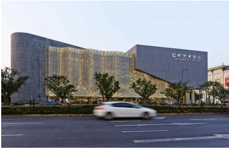
Figure 48: Shanghai Hongqiao Arts Center
