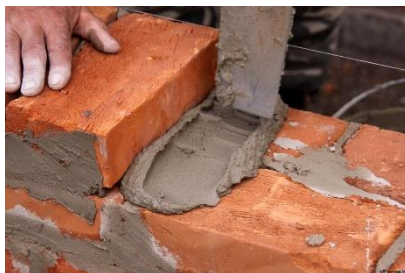
Figure 21: Jointage Source : https://decorexpro.com/cement/izvestkovyj-rastvor/
