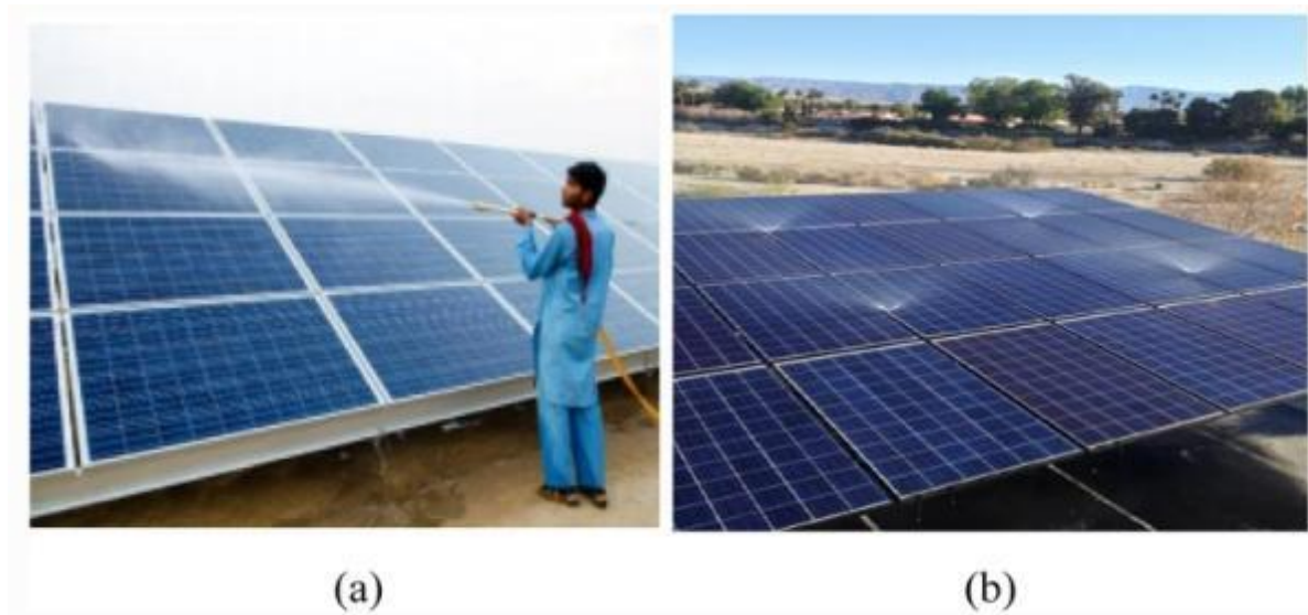
Figure III.4: (a) Water cleaning of PV panels by a labor and (b) using the Heliotex technology [40]
