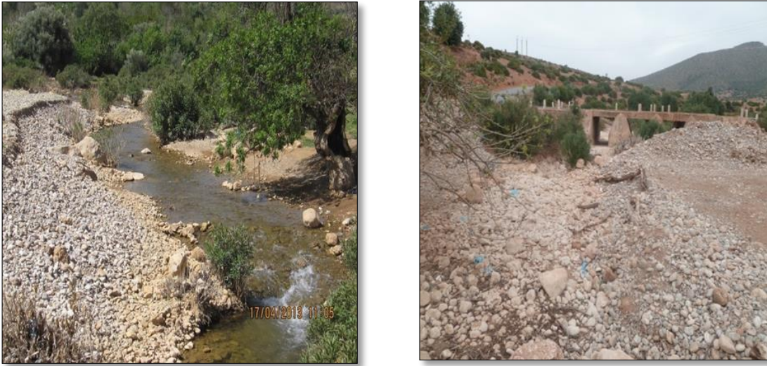
Figure 12 : station de Chouly 2 (Ammouri, 2014).
