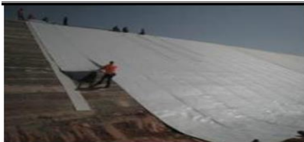
Figure II.13: Installation of membrane (Amara and Dib, 2020)
