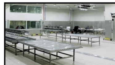
Figure 94 : Hall de production
