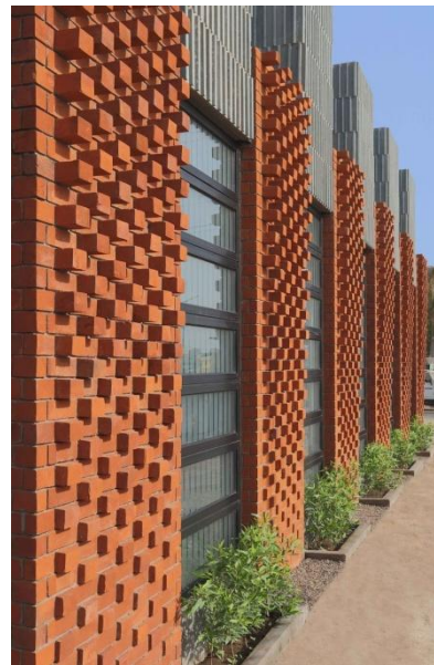
Figure 185. Façade usine Source www.pinterest.com
