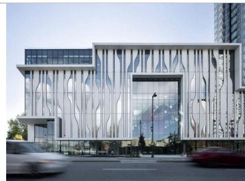
Figure 125 brise soleil verticale
