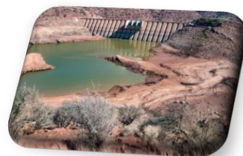
Figure 18 barrage de Beni Bahdel
