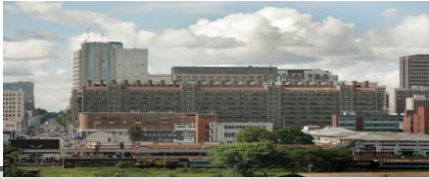
Centre commercial EASTGATE CENTRE à Zimbabwe
