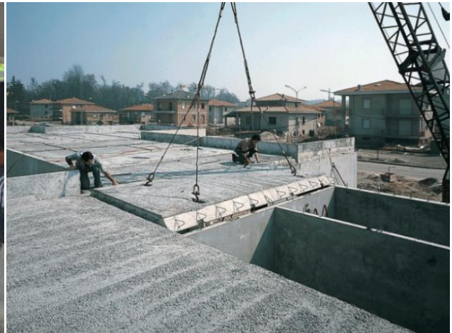
Figure I-9 : Installation de la dalle [6].
