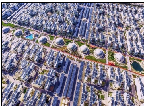
Figure 25 : Eco cité Diamant, Dubaï, Émirats arabes unis Source : https://mid-east.info/diamond-developers-awarded-developer-of-the-year-at-the-mena-green-building-awards-2020/
