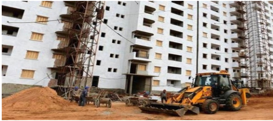
Figure I.1 : Residential construction in Algeria [30].
