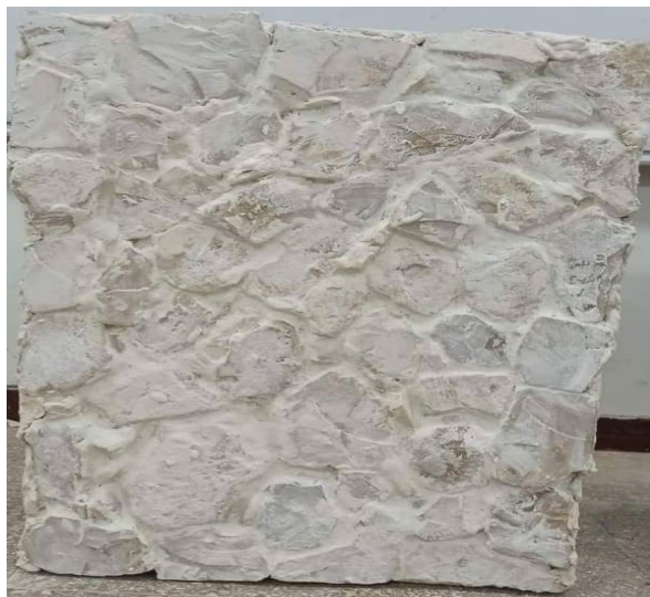
Figure III.4: Brick wall with a PCHCM finishing layer.
