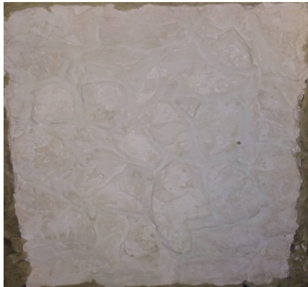
Figure III.3: Brick wall with a Diatomite finishing layer.
