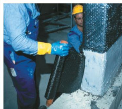
Application de MapeWrap C Uni-AX
