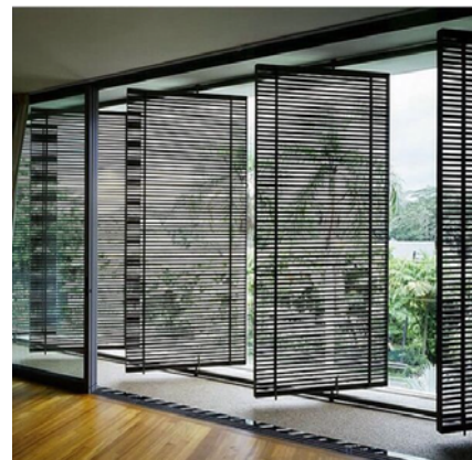
Figure 69. Brise soleil vertical rotatif
