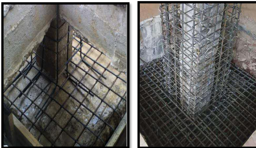
Figure I.13: Renforcement de fondations existantes [9]
