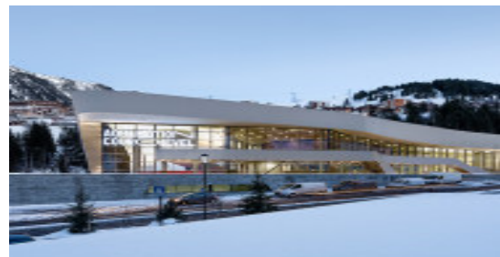
Figure 10 : façade principale (Auer waber)
