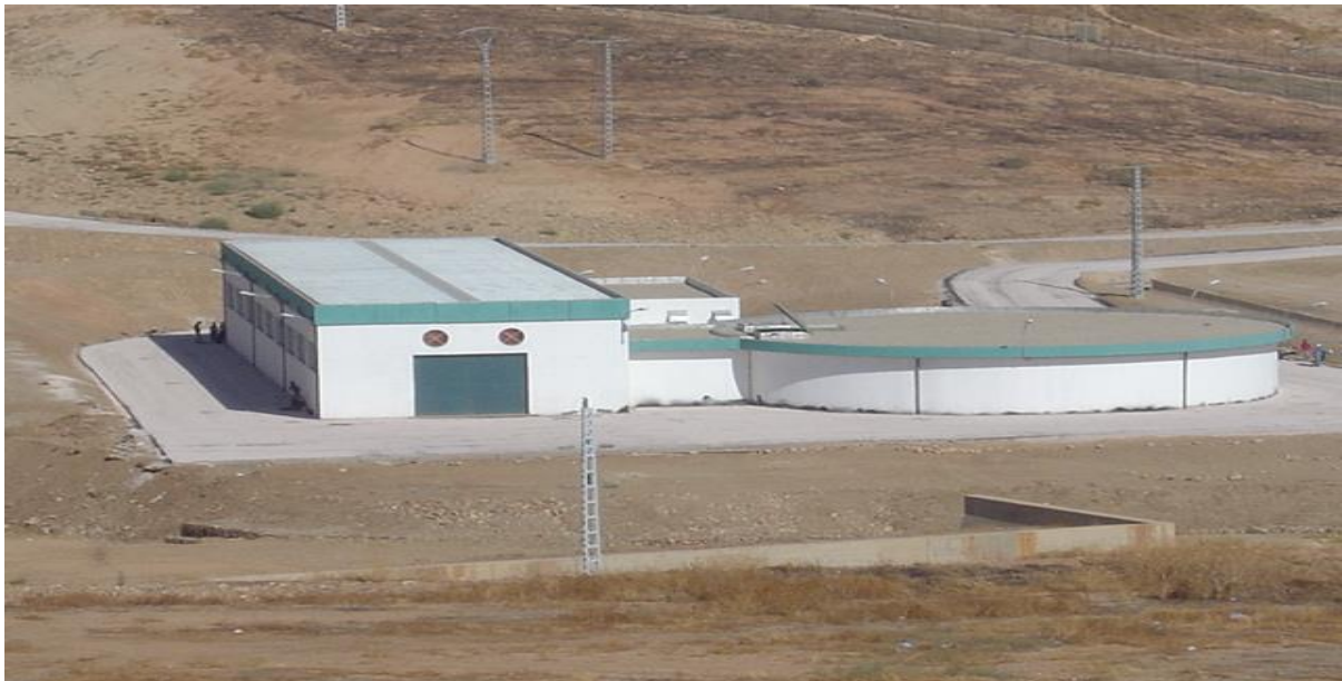
Figure III-17 : Station de pompage (SP1).
