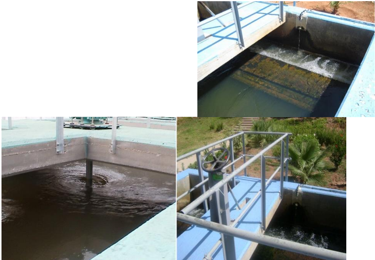
Figure III-7: Bassin de coagulation (Manuel de la station. 2006).
