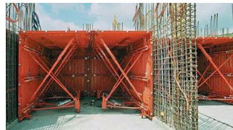
Figure 97. Coffrage tunnel.
