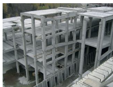
Figure 76. Structure poteau-poutre BA.
